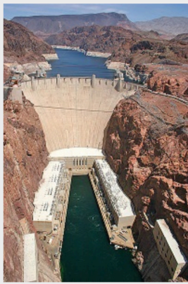
The water pressure pushing on the surface of this dam is an example of a surface force. Image by Curimedia CC-BY-SA 2.0
